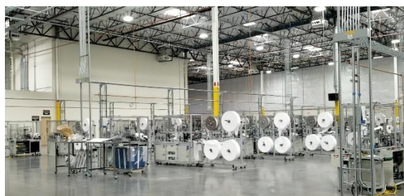
N-95 Mask Manufacturing Plant, 2145 E. 27th Street
